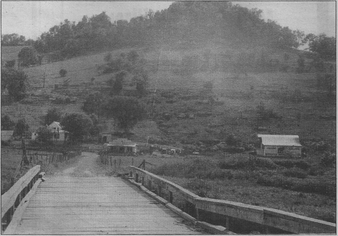
The old bridge at Dry Creek with W.O. Womack's house, barn and store in the background.
